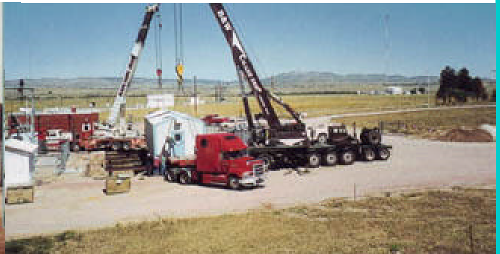
Above and left: Long's latest work at Platte's Guernsey facility was done as a subcontractor to Automation Electronics of Casper, which was installing a totally new electrical control system at the pumping station. Cranes from B&W Crane Service and Black Hawk Crane are seen placing the new control structure, above, while a portion of the maze of electrical lines emanating from the structure is seen at left in trenches excavated by Long's.
