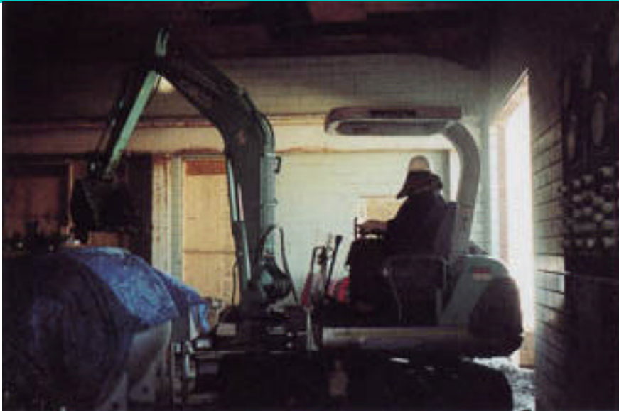
Another advantage of the miniexcavators: they can fit through doorways, facilitating excavation work inside buildings, as here at Platte Pipe Lines Moorefield, Neb., station, where lines serving the unit pumps had to be uncovered and reset.
