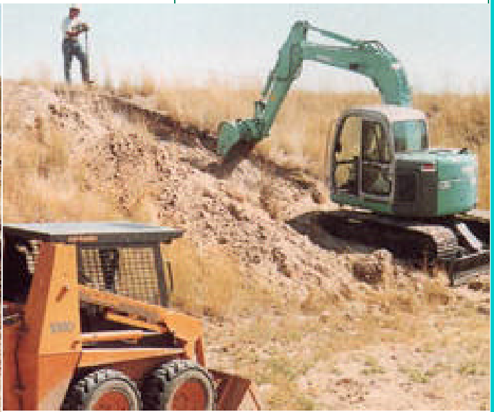
Not all the digging at the Guernsey station was in confined, congested areas. Here, the Kobelco SK70 digs, and later backfills, lengthy trench to carry electrical control cable to adjacent tank farm.
