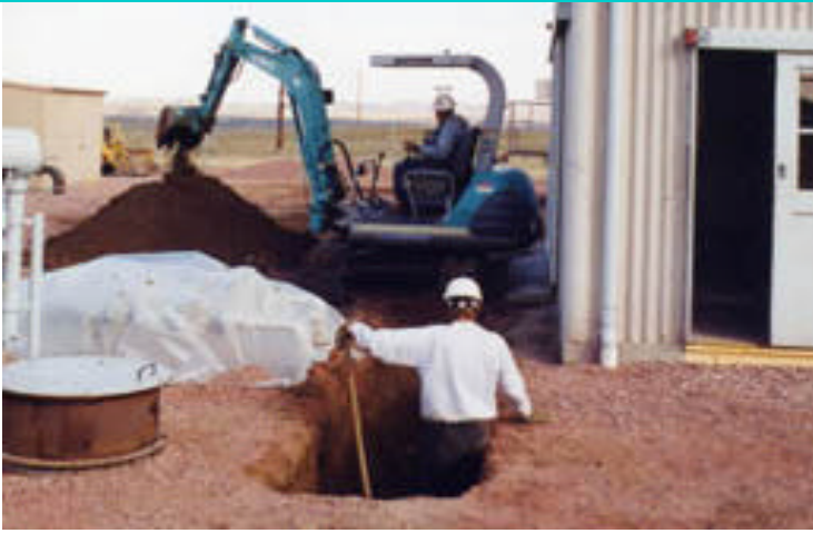
Jerry Long uses one of the Kobelco SK35s to dig a trench alongside a pumphouse at Guernsey. Zero tailswing of the diminutive excavator allows it to work right beside the structure.
