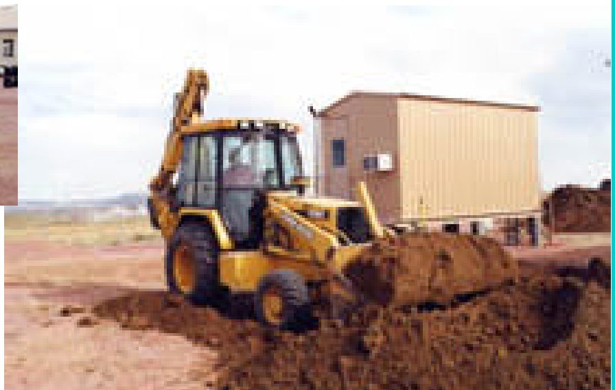
Above and right: In addition to the Kobelco minis, Long's uses a Case 1840 skid-steer loader, seen here removing and stockpiling gravel surfacing, and a John Deere 310D backhoe/loader, seen picking up excavated soil for stockpiling out of the way of the ongoing work.
