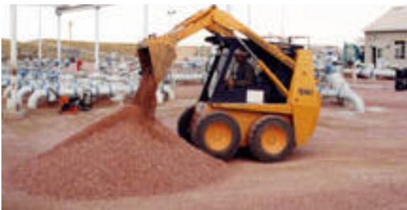
Above and right: In addition to the Kobelco minis, Long's uses a Case 1840 skid-steer loader, seen here removing and stockpiling gravel surfacing, and a John Deere 310D backhoe/loader, seen picking up excavated soil for stockpiling out of the way of the ongoing work.
