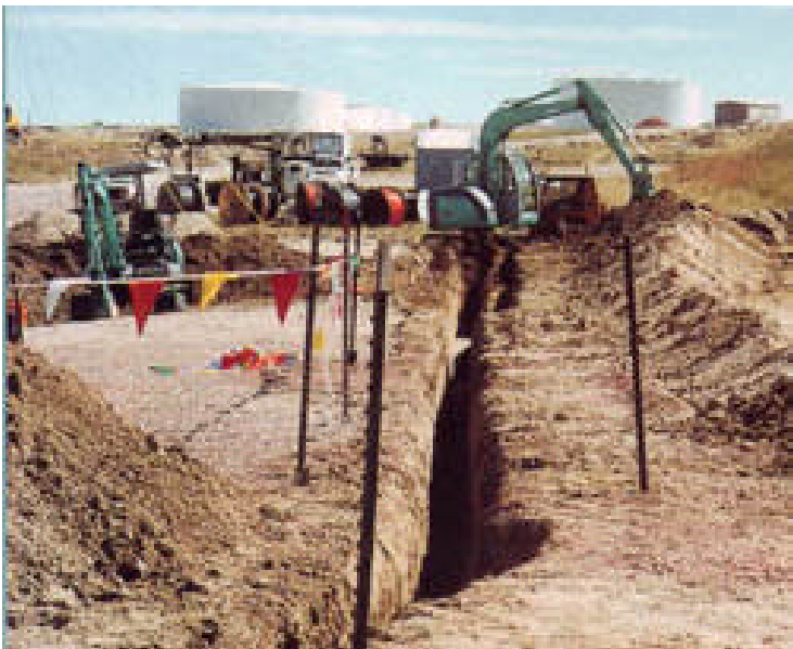
Not all the digging at the Guernsey station was in confined, congested areas. Here, the Kobelco SK70 digs, and later backfills, lengthy trench to carry electrical control cable to adjacent tank farm.
