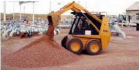
Above and right: In addition to the Kobelco minis, Long's uses a Case 1840 skid-steer loader, seen here removing and stockpiling gravel surfacing, and a John Deere 310D backhoe/loader, seen picking up excavated soil for stockpiling out of the way of the ongoing work.
