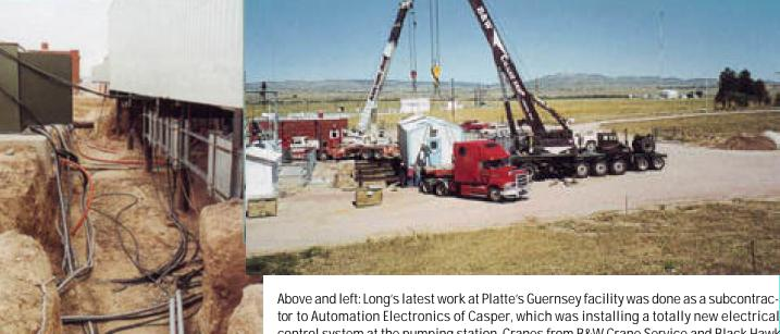
Above and left: Long's latest work at Platte's Guernsey facility was done as a subcontractor to Automation Electronics of Casper, which was installing a totally new electrical control system at the pumping station. Cranes from B&W Crane Service and Black Hawk Crane are seen placing the new control structure, above, while a portion of the maze of electrical lines emanating from the structure is seen at left in trenches excavated by Long's.
