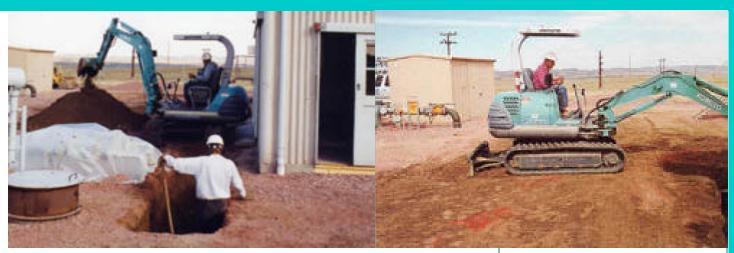
Jerry Long uses one of the Kobelco SK35s to dig a trench alongside a pumphouse at Guernsey. Zero tailswing of the diminutive excavator allows it to work right beside the structure.
