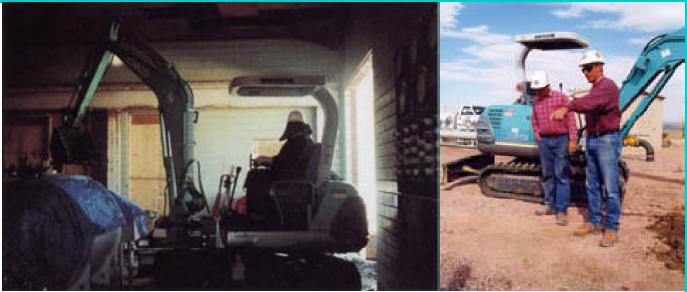
Another advantage of the miniexcavators: they can fit through dodorways, facilitating excavation work inside buildings, as here at Platte Pipe Lines Moorefield, Neb., station, where lines serving the unit pumps had to be uncovered and reset. -- Photo courtesy Long's Excavation
