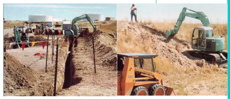
Not all the digging at the Guernsey station was in confined, congested areas. Here, the Kobelco SK70 digs, and later backfills, lengthy trench to carry electrical control cable to adjacent tank farm.
